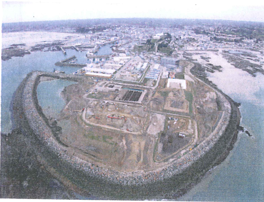
La Collette site viewed from the south: Ash cells are the pits on the right hand side of the site
